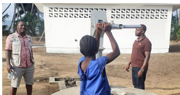
Repair work done on a damaged handpump.
